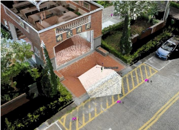
Figure 3. Point Cloud Model after Connection with Yeoh Tiong Lay Garden
